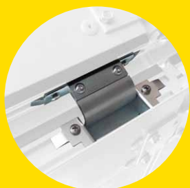
Detail of recessed hinge
